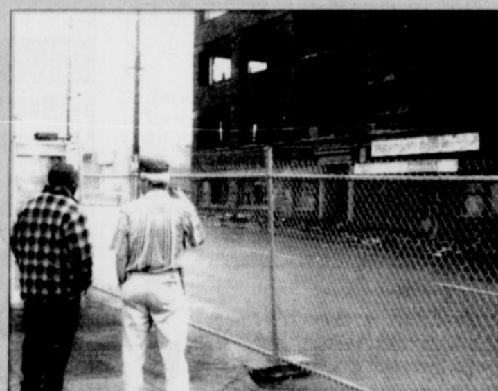
Surveying the damage, area residents look over a gutted warehouse at Northeast Sixth and Davis. The building is in danger of collapsing and has families in an adjacent apartment displaced.
