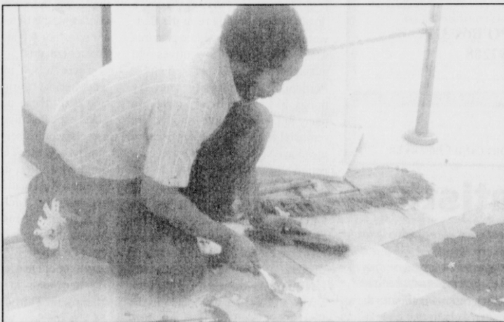
Johnny Olive makes repairs at the new E&M Market.
