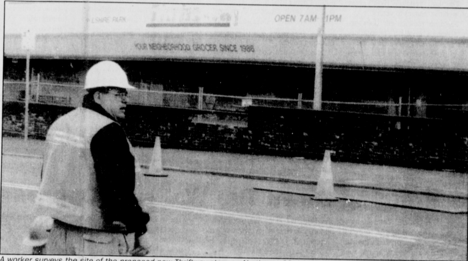
A worker surveys the site of the proposed new Thriftway store on Northeast 33rd Avenue. Photo by Mark Washington.
