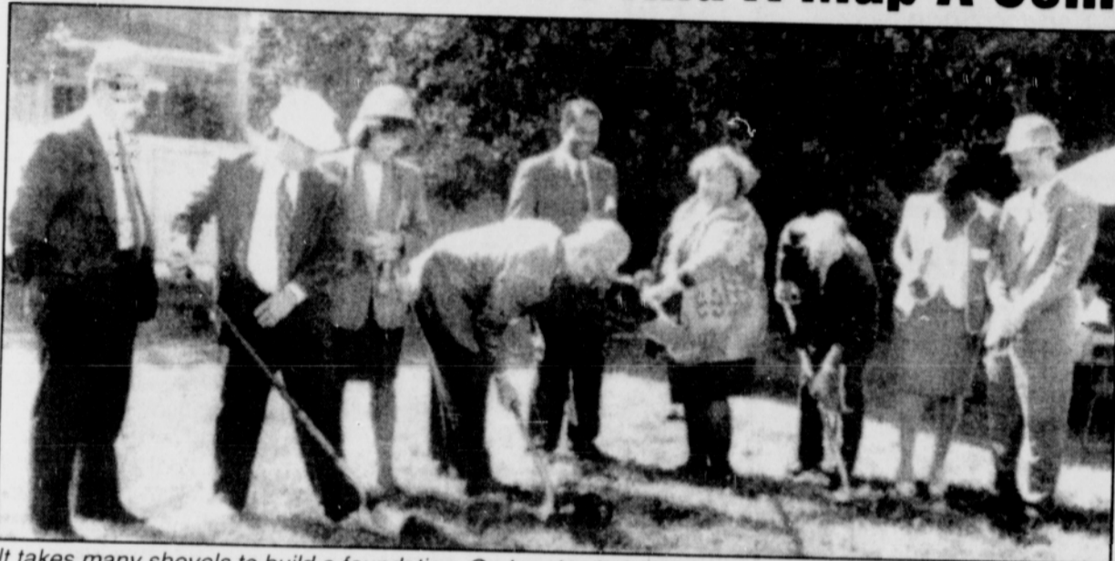
It takes many shovels to build a foundation. On hand to help NECDC's Walnut Park townhouses get off to a good start are Brian Stewart (Washington Mutual), Scott Christensen (Key Bank), Karen Tolvstad (US Bank), Jim Taylor (Portland Trail Blazers), NECDC board member George Richards, Shiela Holden (Neighborhood Association), Bill Van Vliet (FIB), NECDC Executive Jaki Walker, and Dick Hanlin (Boys and Girls Club).
