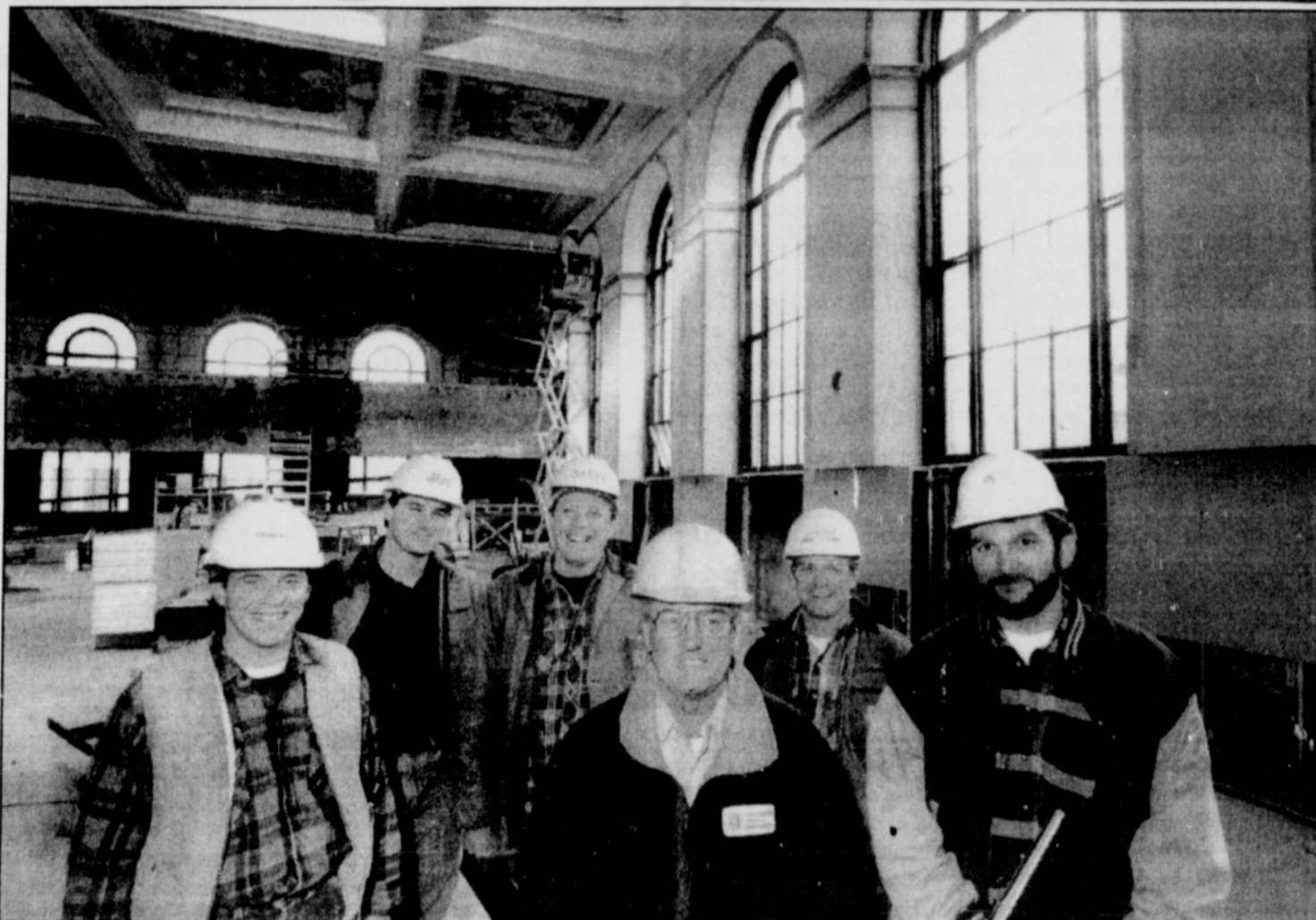
Renovation of the historic downtown Multnomah County Central Library has included work by Dave Schwab (from left) Joe Squires, Steve Johnston, Barry Woods, Bill Bader and Steve Gourde, members of National Electrical Contractors Association and International Brotherhood of Electrical Workers, Local 48.
