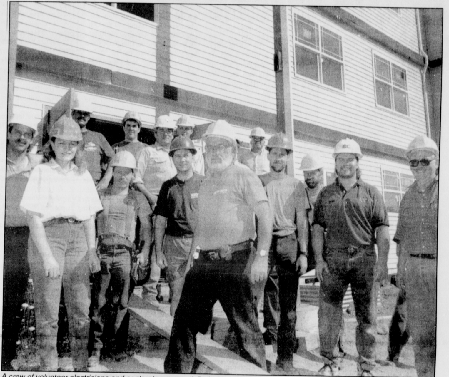
A crew of volunteer electricians and contractors are satisfied with a job well done as they wire the new Open House Ministries homeless shelter.
