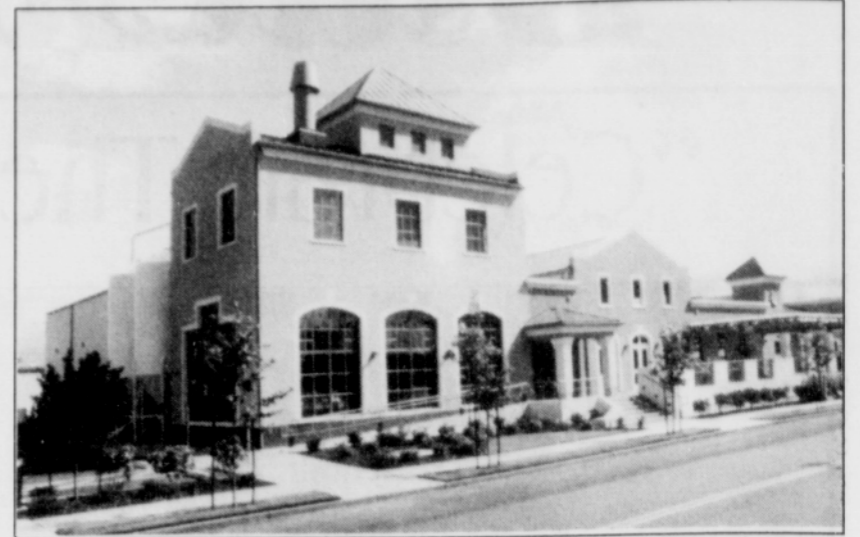
Portland Brewing Company continued a 447-year tradition of German brewing when it brought on-line at its new brewer classic copper brewing equipment purchased from the Sixenbrau Brewery in Nordlingen, Germany. The new brewery, funded in part by the first microbrewery public offering in the State of Oregon, increases the company's capacity and will soon feature the new "Brewhouse Taproom" for sampling its fine, hand-crafted beers.
