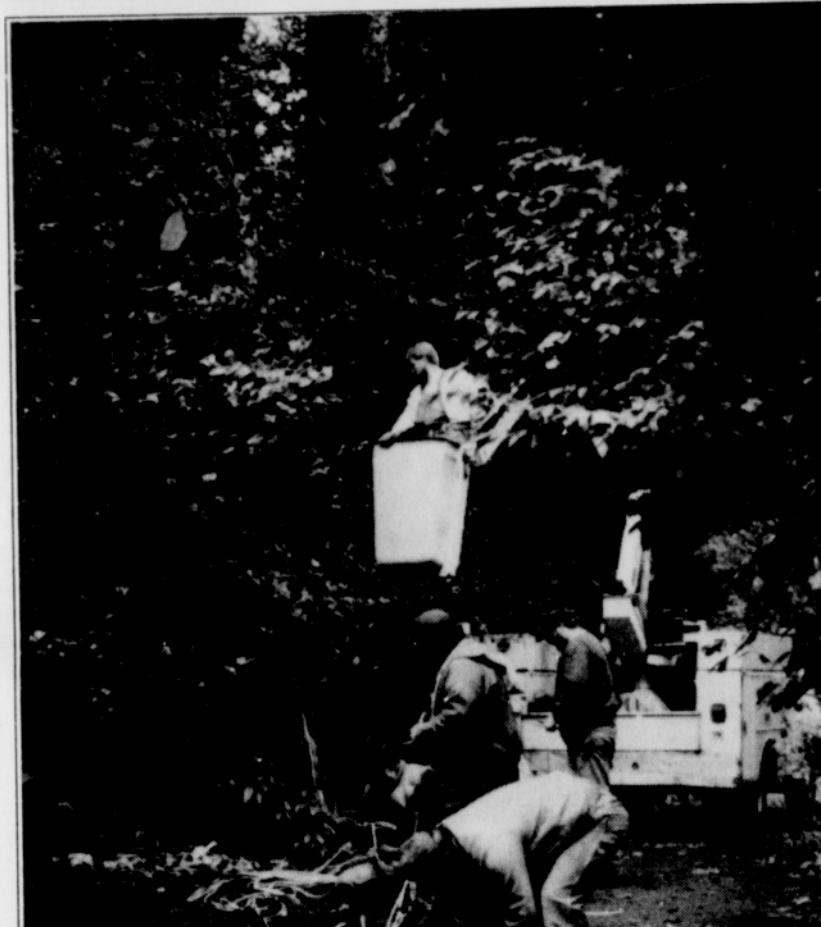
The 28 volunteers from Local 48 devoted their Saturday, prior to Thanksgiving, providing the electrical work needed to generate temporary power for over 50,000 lights
