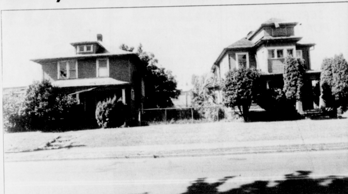
Previously abandoned houses to be renovated for the Neighborhood Health Clinics, Inc.
