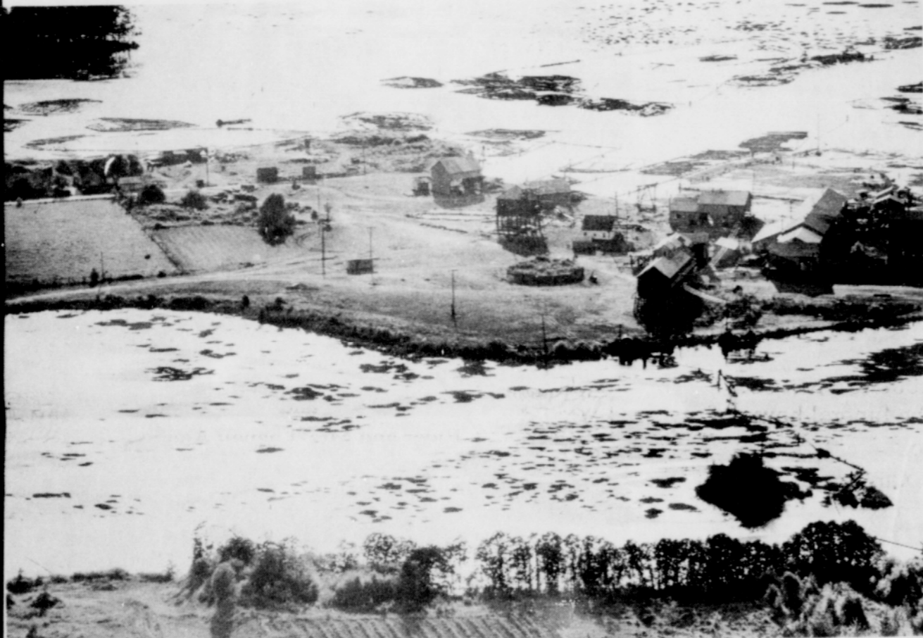
Aerial overview of the flood rushing thru Vanport.
