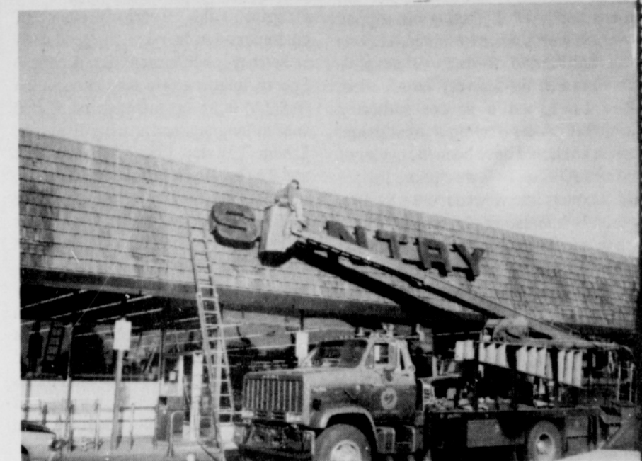
Workers Install Sign
