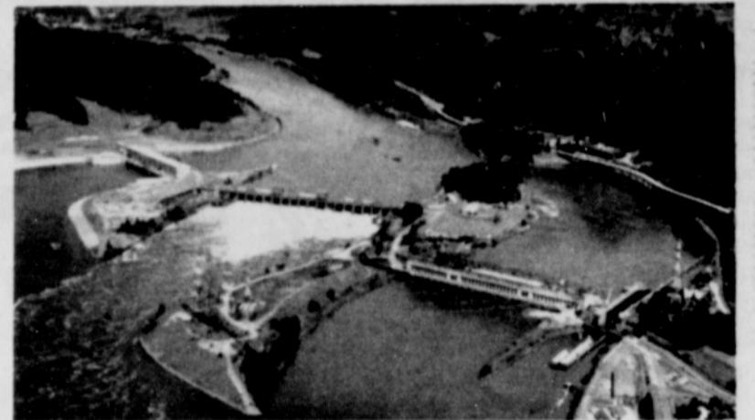
October 1983 - The entire Bonneville project stretches across the Northwest's largest river, the Columbia, between Washington and Oregon. The original project, the lock and dam seen at right, and the spillway, center, was built during the Depression. The Second Powerhouse is left of the spillway with newly created Cascades Island between. Together the two will produce an annual average of 6.1 billion kwh. The Second Powerhouse will be dedicated June 1, 1983.
