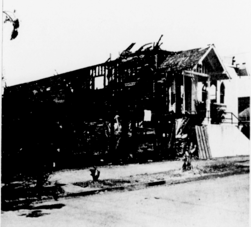
Providence Baptist Church and an apartment building on Failing and Garfield were burned as a result of arson. Anyone seeing any cars or people in the area at around 4:00 a.m., Friday are asked to call the arson department, 248-4363.
