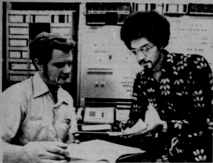
SETTING UP NEW SYSTEM — Pacific Northwest Bell technicians Dave Harris (left) and Rich Nelson consult on testing of new computerized equipment that will serve PNB customers in North and Northeast Portland starting November 4th. New $2.5 million Electronic Switching System will serve PNB customers who have phone numbers with 285 and 289 prefixes.
