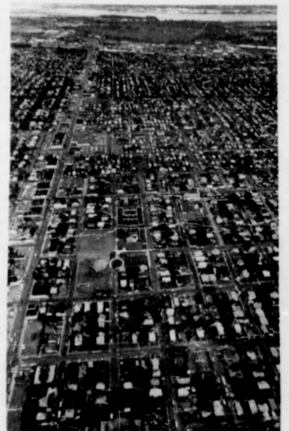
Looking north on Union Avenue.
