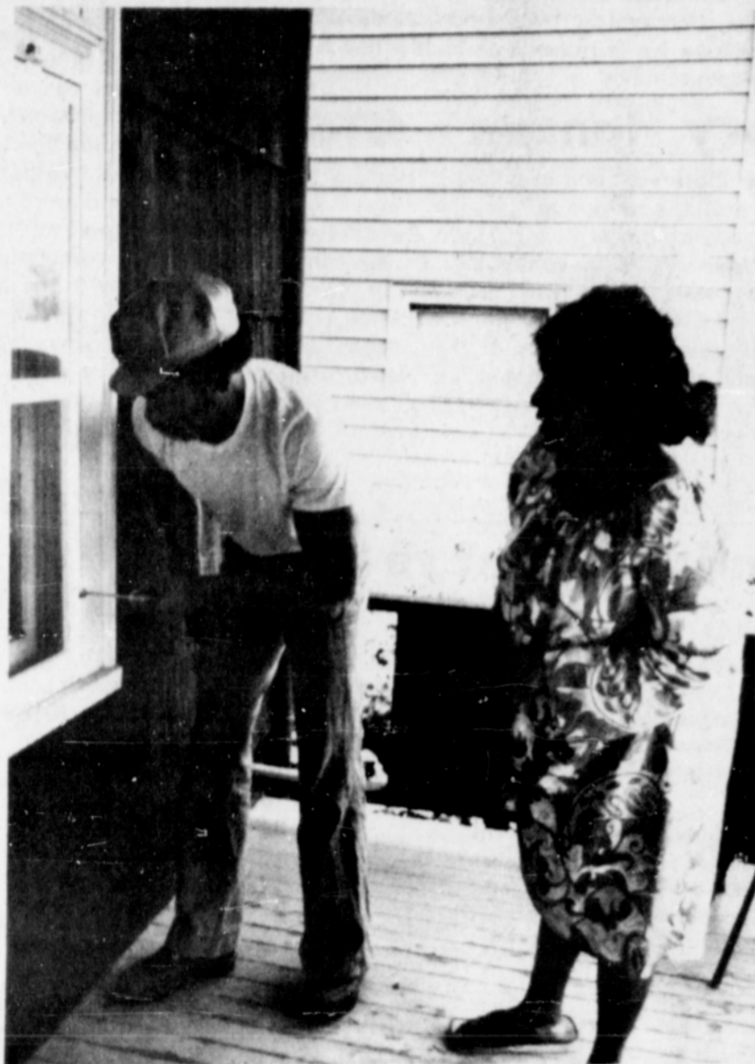
Mrs. Geneva Blake watches as window is repaired by CREP worker.
