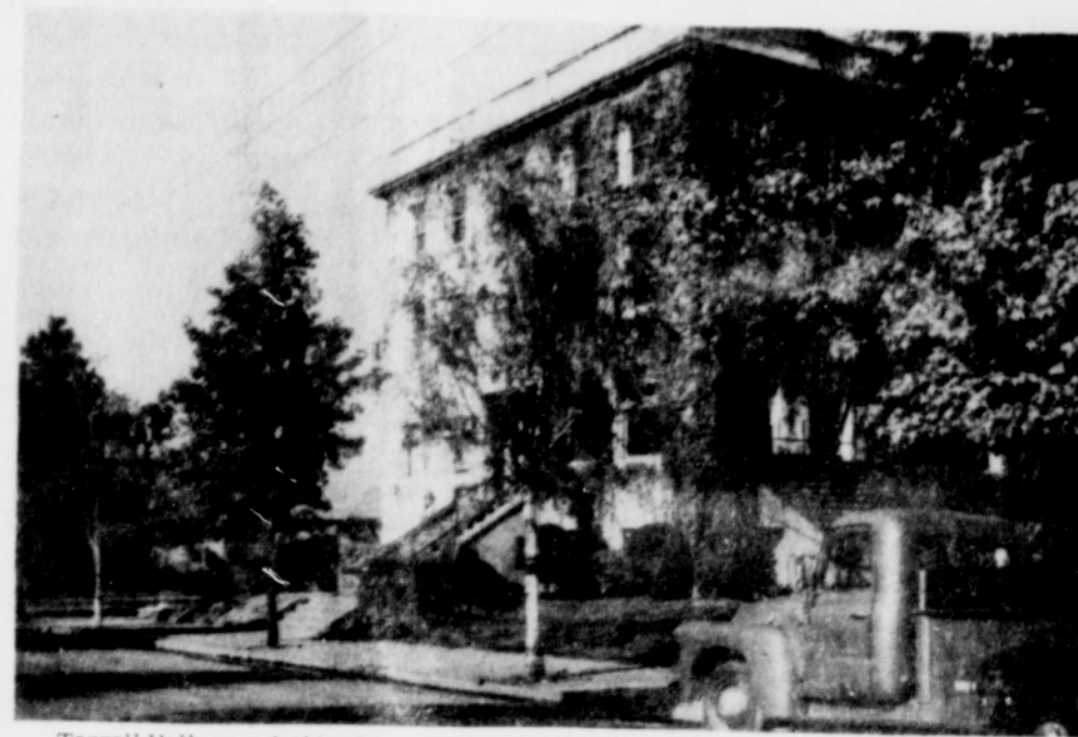
Terrell Hall, an existing structure being remodeled for vocational classrooms.
