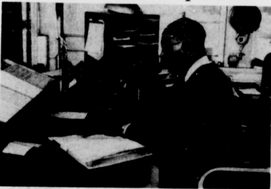
MR. HERNDON concentrates on the controls which manipulate the switches and signals.
