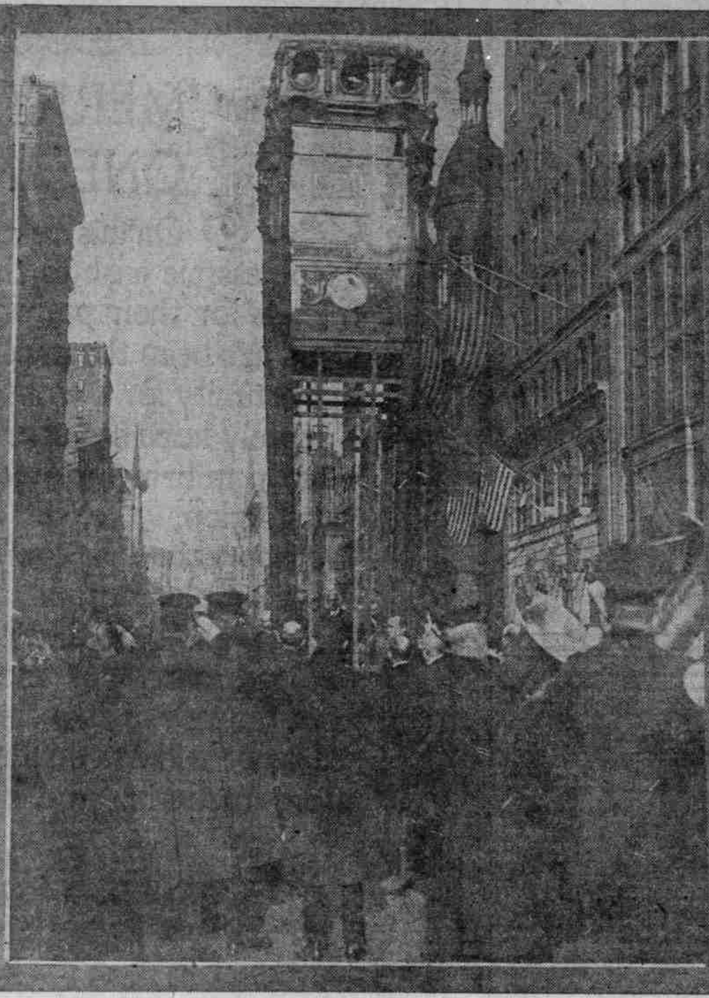
MASTER TOWER AT FORTY-SECOND STREET AND FIFTH AVENUE. This picture shows—just after it was unveiled—the master tower at Forty-second street, controlling all traffic in the business section of Fifth avenue—first of the seven new bronze structures which will replace all of the present unsightly towers of wood and iron on Fifth avenue before the first of the year.
