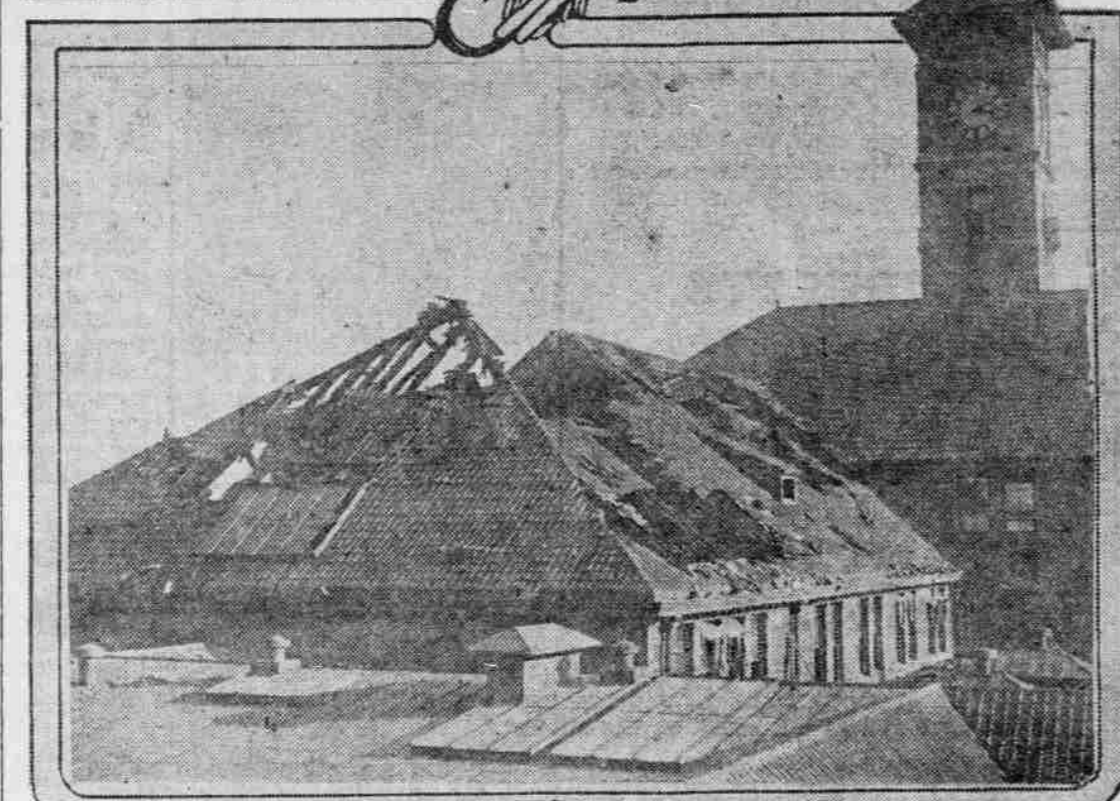
Lower—Another view of the west wing taken from the street in front of the depot showing damage to the second floor.
