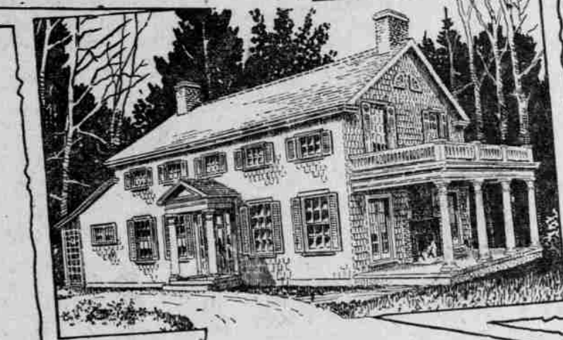
Dunthorpe home of H. G. Conover, Edgemoor Road south of Greenwood Road; Fenner Mfg. Co., architects.
