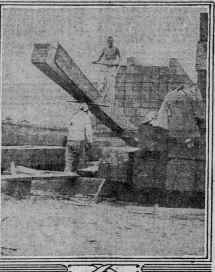
Hand-sawing Oregon Timber at Tientsin.
