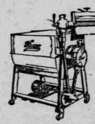
Is the wood cylinder for home use. For over 10 years this cylinder has been built of selected white maple for use in the Thor washer. Experiments with every kind of material,
