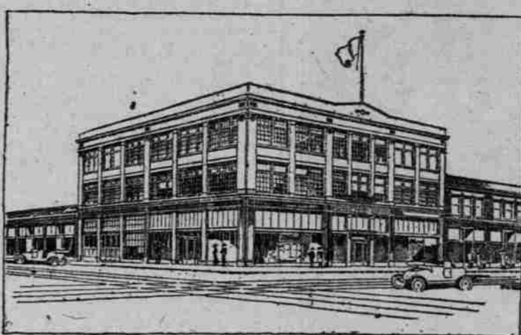
Our New Home Now Under Construction at Grand Avenue and Hawthorne
