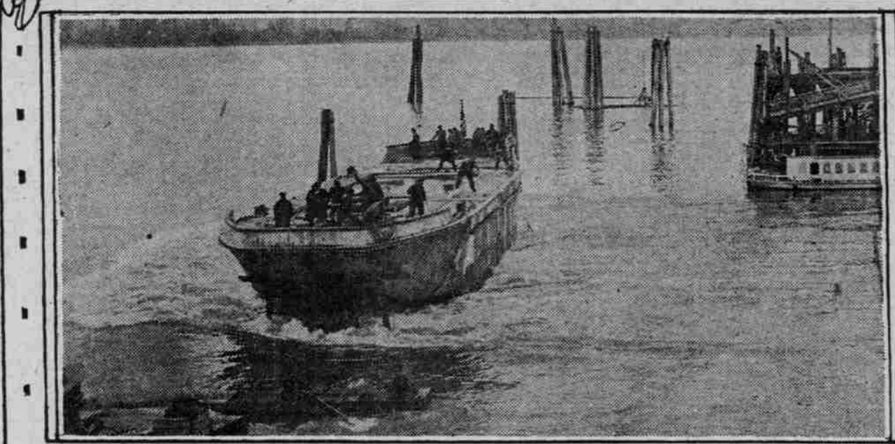
Launching a Concrete 100ft. Ship.
