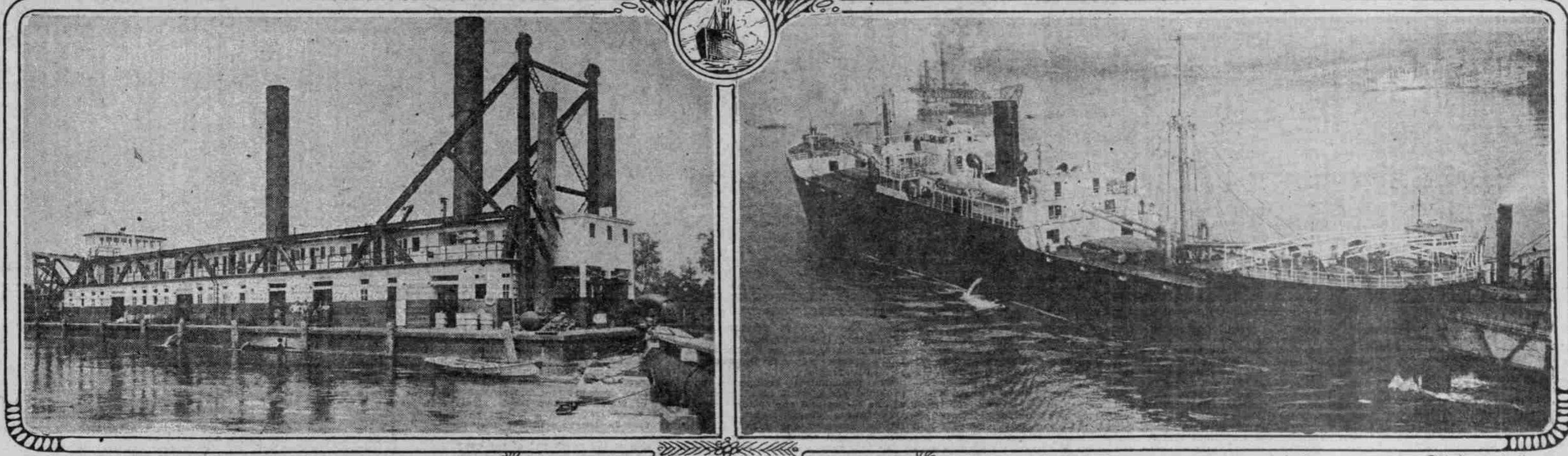
Dredge Willamette at North Portland Harbor
