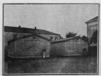
Well painted as it is, this "Portable" does not reveal the flimsiness of its construction. It is sheeted with boards, lined with paper and has a tarred roof.
