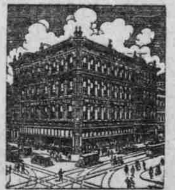
WOOLEN MILL BUILDING
