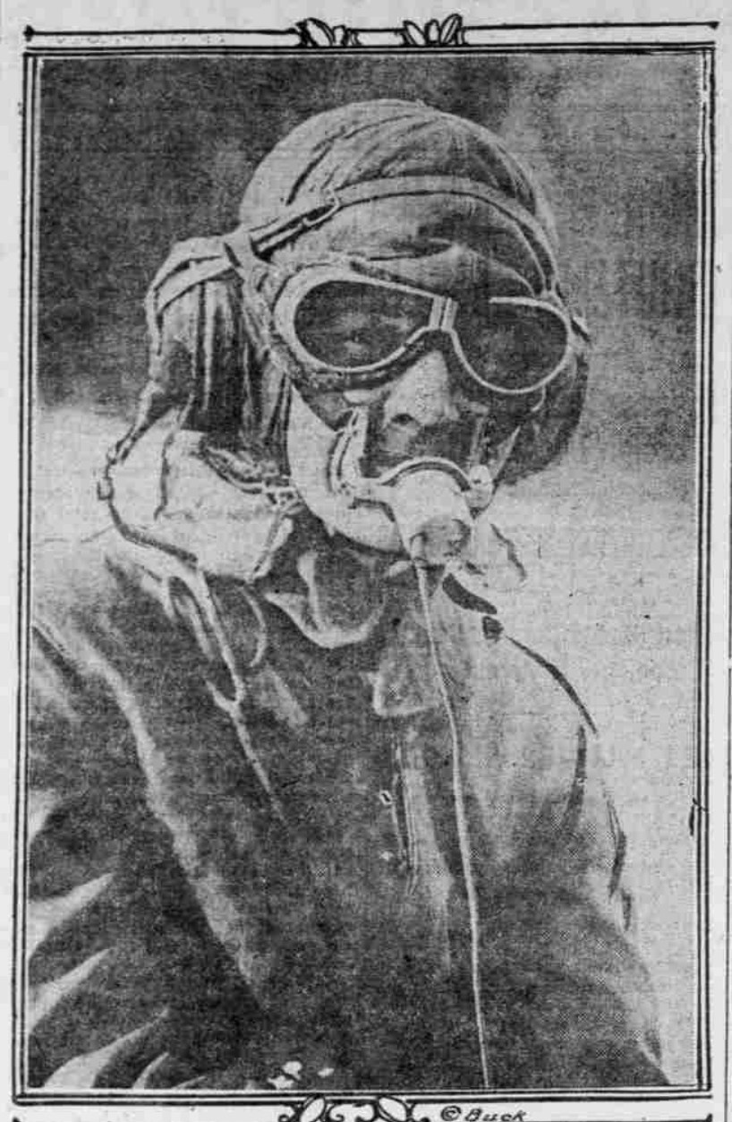
Secretary of the Navy Daniels, on March 12, conversed with the aeroplane of Ensign Harry Sadeauwater, in flight 150 miles away. This conversation, carried on via wireless telephone, was from the secretary's desk to the plane at sea, 150 miles away, and broke all former records, which were from 40 to 50 miles. Our photo shows the wonderful apparatus used on the plane, which has done much toward making wireless telephony an everyday possibility.
