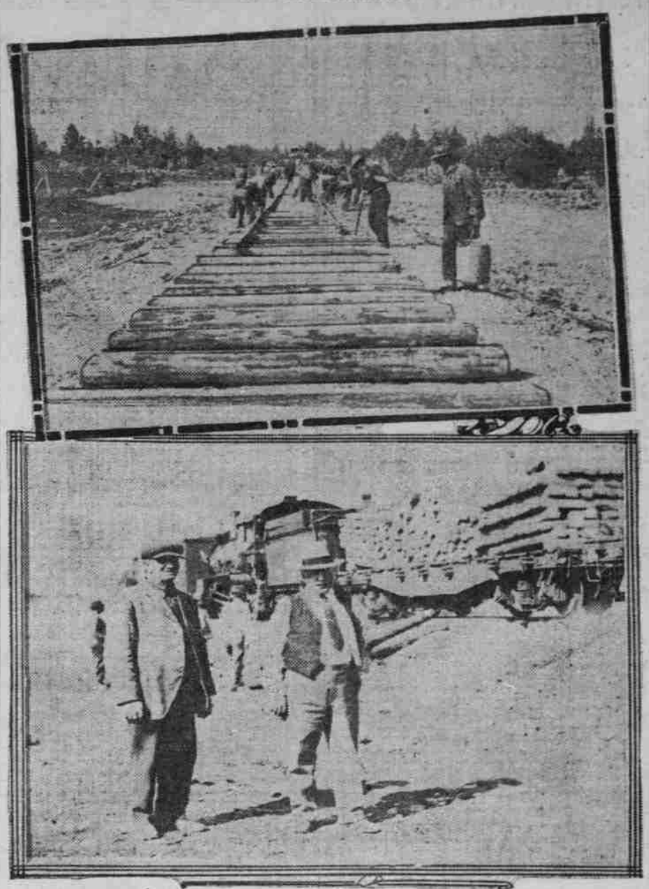
Top, Track Laying in Progress. Below, Mayor D. F. Stewart (Left), of Prineville, and P. L. Gogerty, Superintendent of Construction, Standing by Train on Finished Portion of Track.
