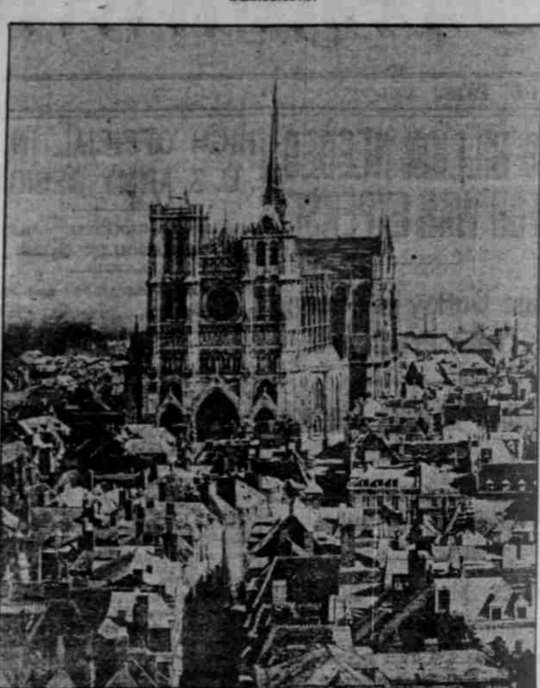
CATHEDRAL OF AMIENS, DAMAGED BY SHELLFIRE.
