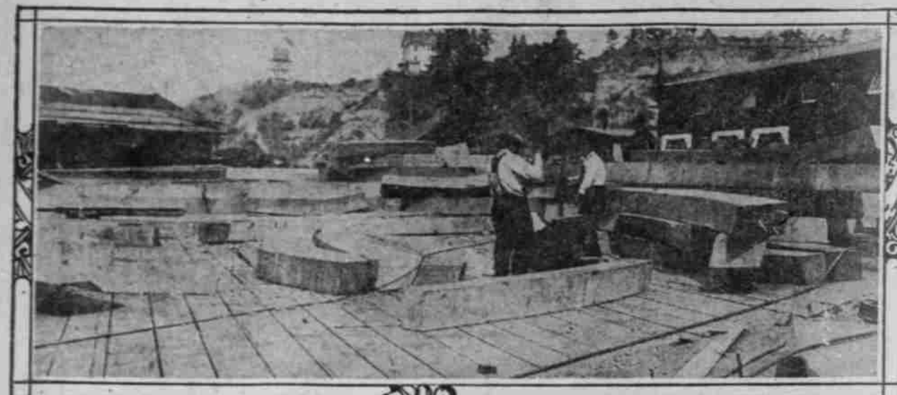
Timbers Shaped for First Wooden Vessel of Present Shipbuilding Program.
