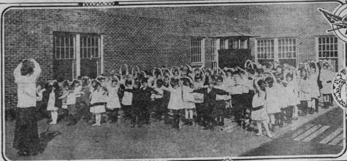
Roof Playground at Couch School.
