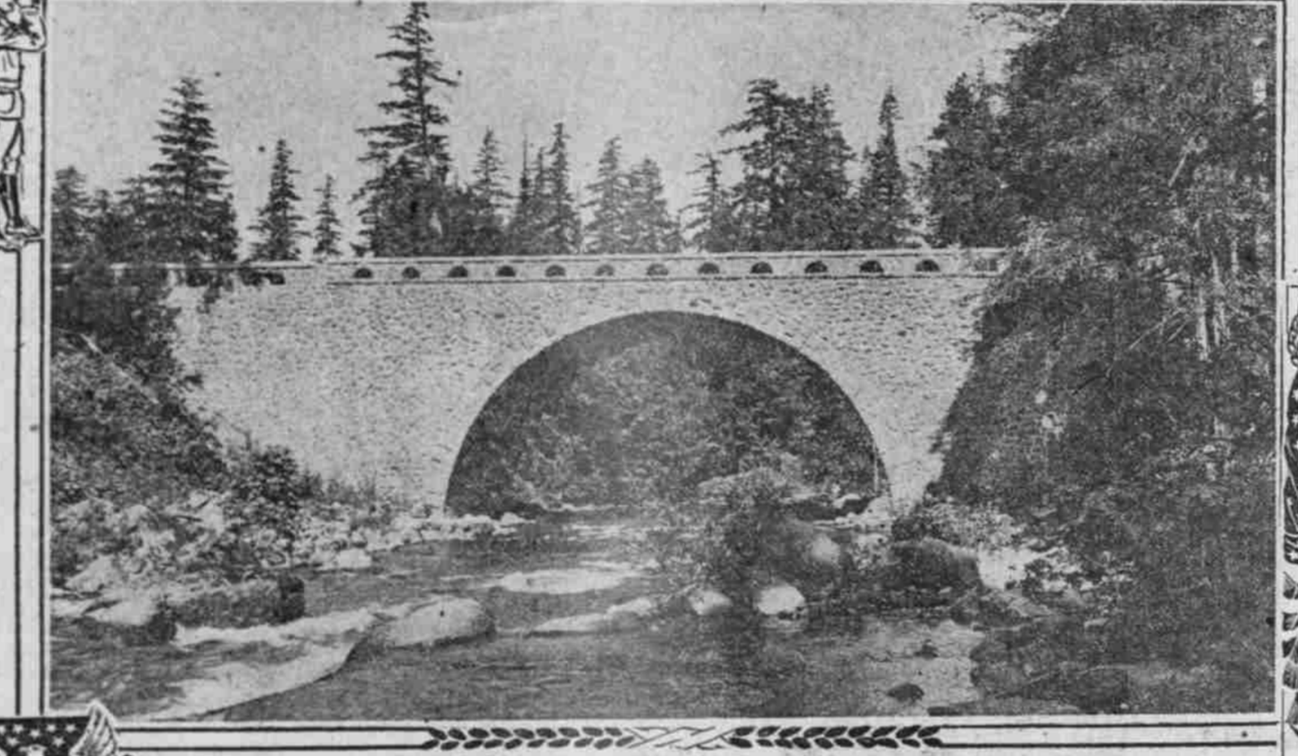
Moffatt Creek Bridge PHOTO GIFFORD & PRENTISS
