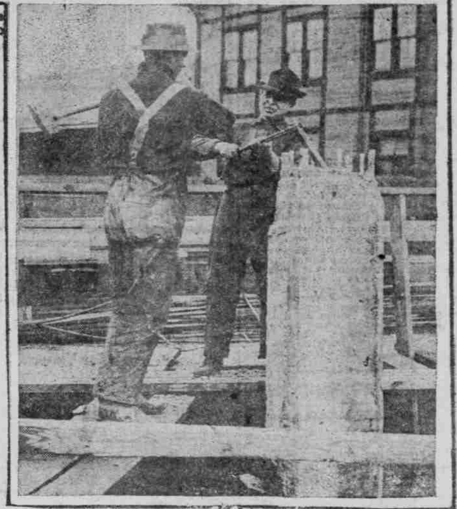
Top, Left to Right—C. C. Holloway, Superintendent of Construction for Government; Grant Fee, Contractor in Charge of the Construction Work; T. Ronneberg, Architect. Bottom—Workmen Trimming Off Top of Concrete Pile That Has Been Driven Down 35 Feet at Hoyt and Gilsan Streets.
