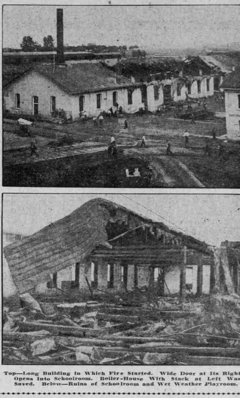
Top—Long Building in Which Fire Started. Wide Door at Its Right Opens Into Schoolroom. Boiler-Room with Stack at Left Was Saved. Below—Ruins of Schoolroom and Wet Weather Playroom.
