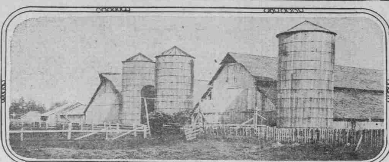
150 Ton Silos and Cow Barns.
