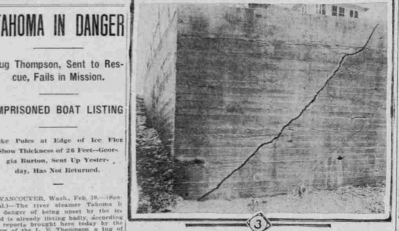
(2) Slide at First and Grove Streets, Which Has Taken Out Half of First Street. (3) View at Rear of Beautiful $12,000 Home of W. C. Lawrence on Montgomery Drive, Which Has Moved More Than a Foot Out of Place by Movement of Ground Toward an Impending Slide. Behind the Camera is a Gully Several Hundred Feet Deep With Large Cracks Developing and Showing the Retaining Wall in Rear of Lawrence Home, Showing One of Many Slowly Widening Cracks. This Wall Has Moved Nine Inches Out of Place.
