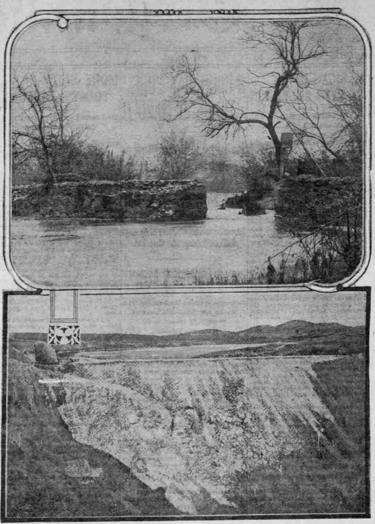
TOP—OLD DAM BUILT IN 1769 BY FRANCISCAN FATHERS ON SAN DIEGO RIVER, 12 MILES FROM SAN DIEGO. BELOW—OTAY DAM.
