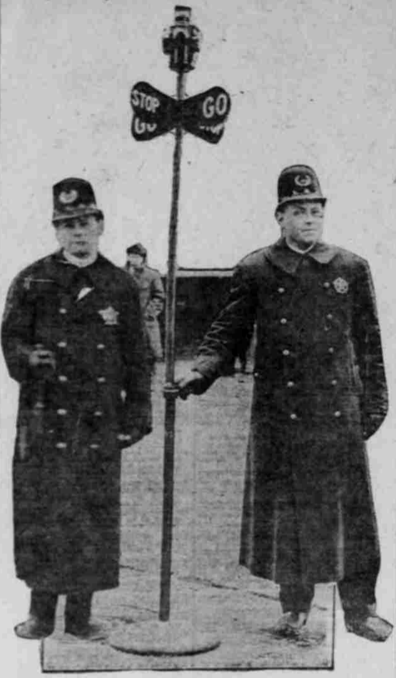
LEFT—J. L. CORDES AND J. J. SAUL, AND AUTOMATIC TRAFFIC SIGN, ERECTED BY MR. SAUL.
