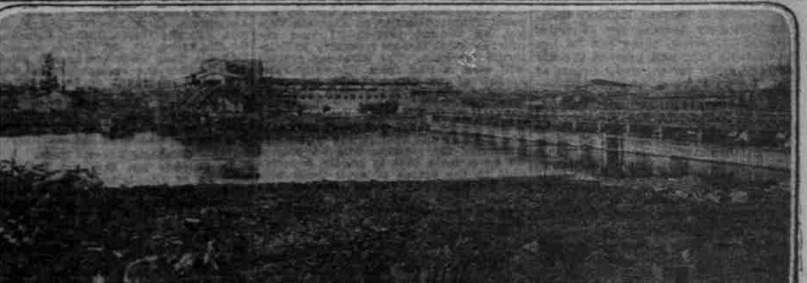
General View of Shevlin Plant Under Construction at Bend.
