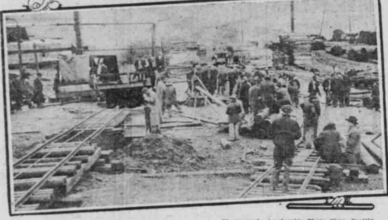
TOP—TAKING DEAD FROM MINE. BELOW—SCENE AT MOUTH OF MINE.
