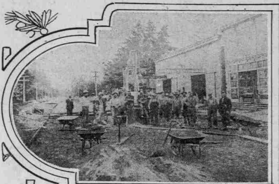
Gang at Work Paving Street in Elma.
