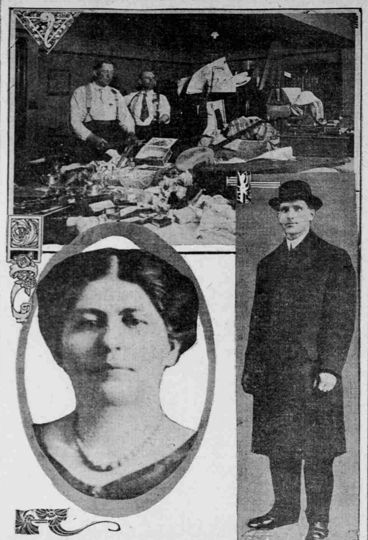
Top-View at Police Headquarters Where Loot of H. G. Hanson Is Held, Showing Detectives La Salle (Left) and Leonard, Whose Efforts Led to the Burglar's Capture. Left—Mrs. Inga Malm, Alleged to Be the Accomplice of Hanson. Right—H. G. Hanson.
