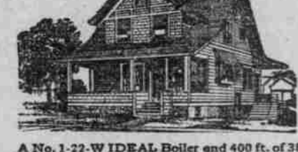
A No. 1-22-W IDEAL Boiler and 400 ft. of 3/8-in. AMERICAN Radiators costing the owner $190 were used to heat this cottage.
