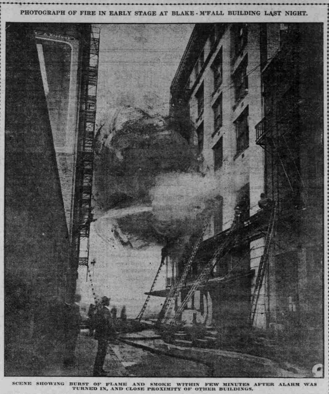
PHOTOGRAPH OF FIRE IN EARLY STAGE AT BLAKE-MCFALL BUILDING LAST NIGHT. SCENE SHOWING BURST OF FLAME AND SMOKE WITHIN FEW MINUTES AFTER ALARM WAS TURNED IN, AND CLOSE PROXIMITY OF OTHER BUILDINGS.
