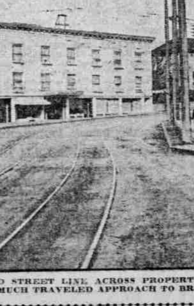
DOTTED LINE SHOWS PROPOSED STREET LINE ACROSS PROPERTY NOW FORMING DANGEROUS OBSTRUCTION IN MUCH TRAVELED APPROACH TO BROADWAY BRIDGE.
