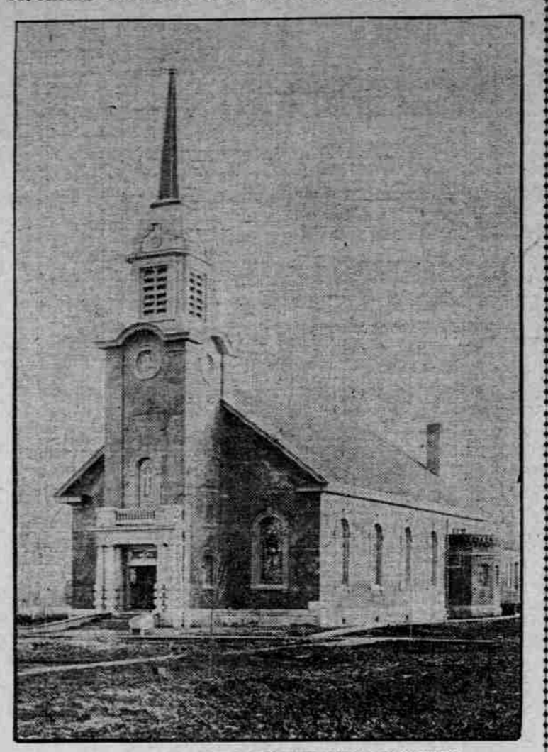
NEW EDIFICE THAT HAS JUST BEEN COMPLETED. M'MINNVILLE, Or., Jan. 20.—(Special.)—The new St. James Catholic Church was dedicated here Sunday by Archbishop Christie, assisted by Father Charles Raymond, of McMinnville, and Father O'Hara, of Astoria. The cornerstone was laid July 19 last year. The temple has a seating capacity of more than 500.
