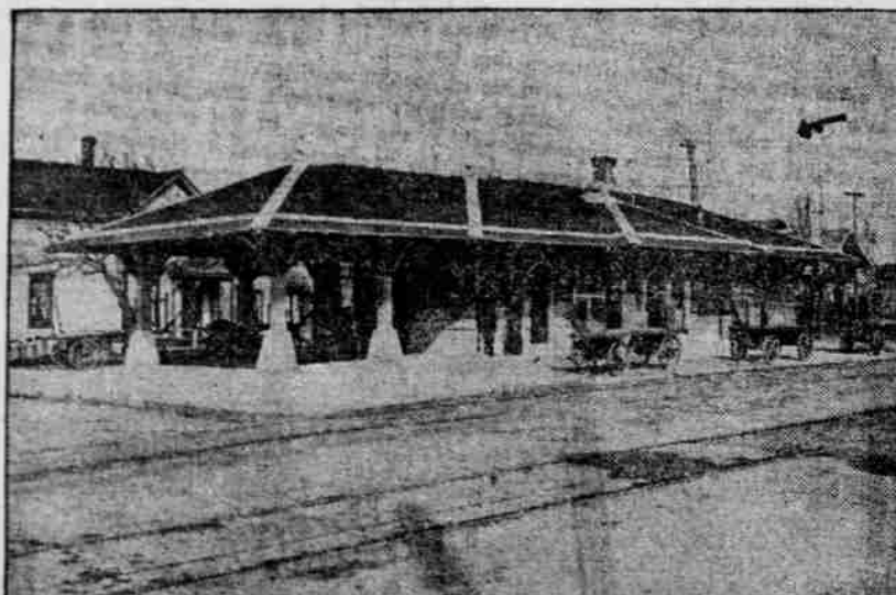
Southern Pacific Modern Passenger Station, McMinnville, Ore.
