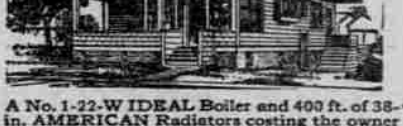
A No. 1-22-W IDEAL Boiler and 400 ft. of 38-in. AMERICAN Radiators costing the owner $150, were used to heat this cottage. At this price the goods can be bought of any reputable, competent fitter. The cost does not include costs of labor, pipe, valves, freight, etc., which vary according to climatic and other conditions.
